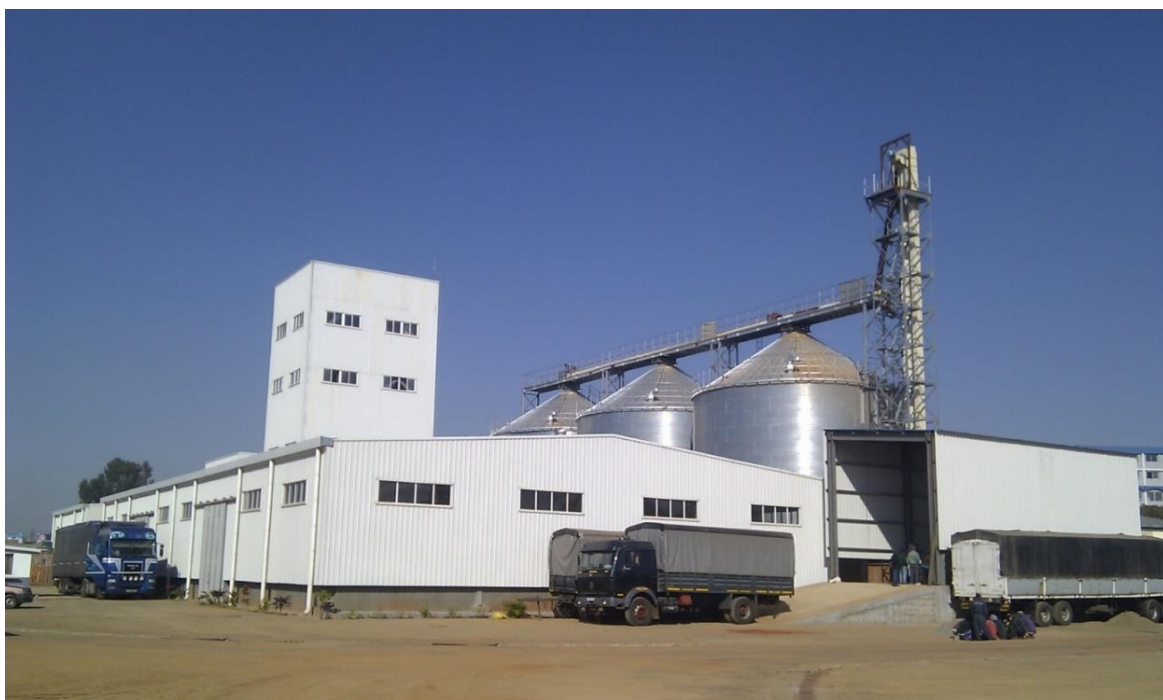
Photo: Groupe SMTP’s animal feed mill, construction completed in 2010 by FAMSUN.
